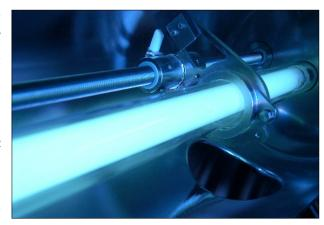
Ozone gas is also sucked through the exhaust ducts breaking down any grease that has collected deeper inside the ductwork. Another benefit is that the Ozonolysis process has the effect of deodorizing the exhaust air- an increasing requirement in many countries
